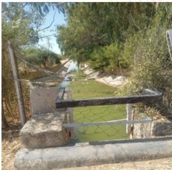
Fig. 1: Canal outlet structure in the arid zone
